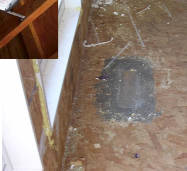
COVERING DUCT OPENINGS DURING CONSTRUCTION
