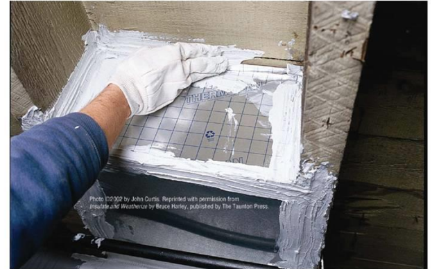
SEALING WITH MASTIC
