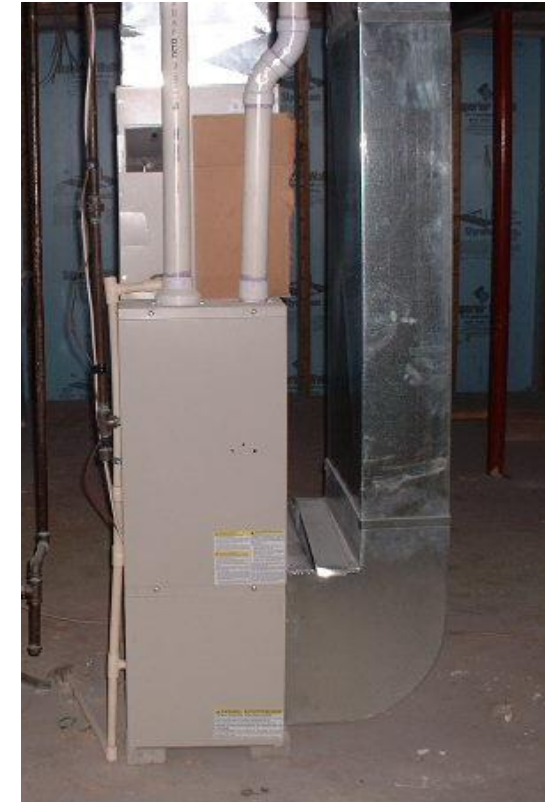
DIRECT VENTED FURNACE
