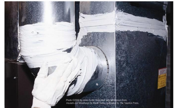
SEALING WITH MASTIC
