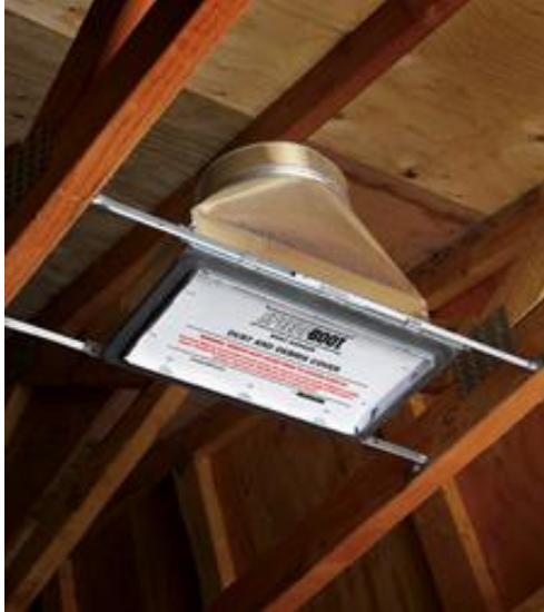
COVERING DUCT OPENINGS DURING CONSTRUCTION
